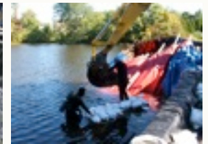
Divers worked in the water to construct portions of the ladder
