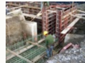
Construction of the denil fish ladder- setting the concrete forms
