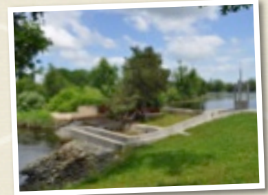
Kickemuit River Fish Ladder & Dam.
